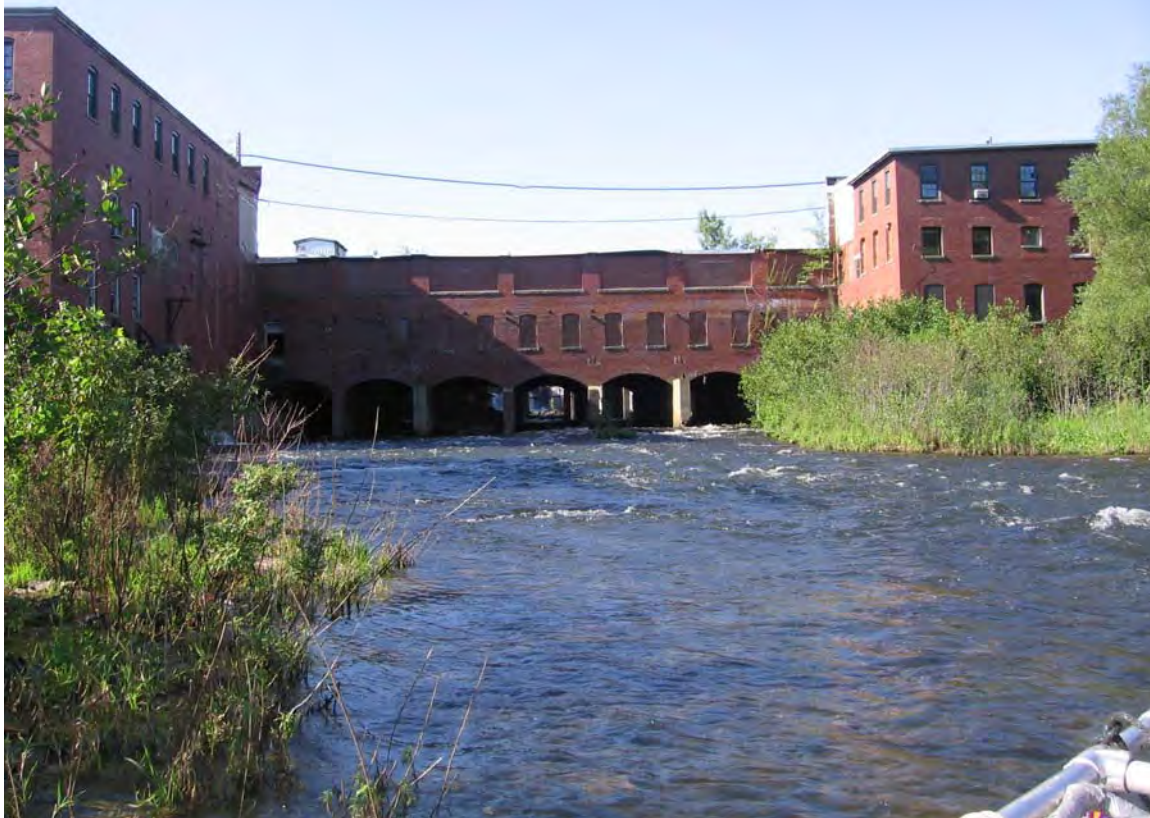
Plate 1. Upper: Lower Presumpscot Falls looking downstream (August 2006). Lower: Looking upstream at a portion of the Cumberland Mills Dam and SAPPI facility (August 2006).
